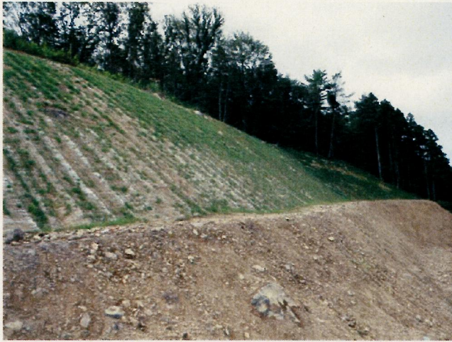
①法面緑化状況 (採石場の南端)
